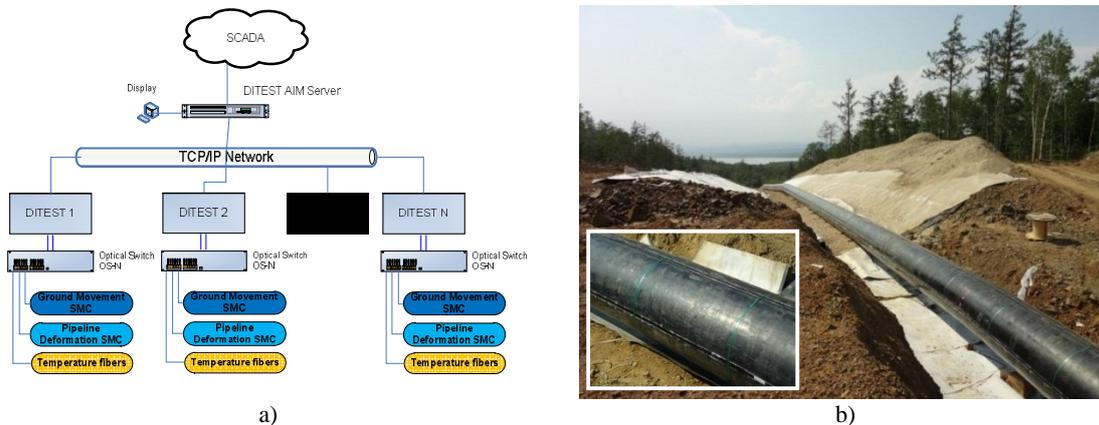
Figure 2. a) Monitoring architecture featuring multiple DITEST interrogator and TCP/IP communication to a central AIM server for event monitoring and alarming and b) trench featuring a section of pipeline instrumented with 3 strain sensors for 3D deformation with close view (inset).
